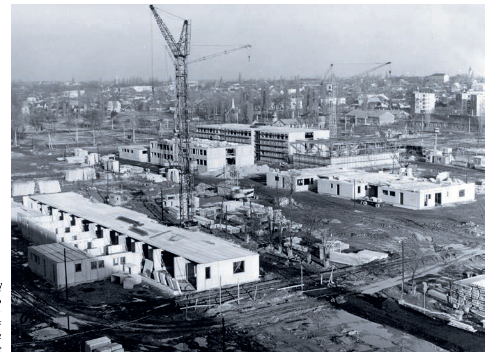
Épül a Havanna-lakótelep Construction works of the Havanna housing estate
